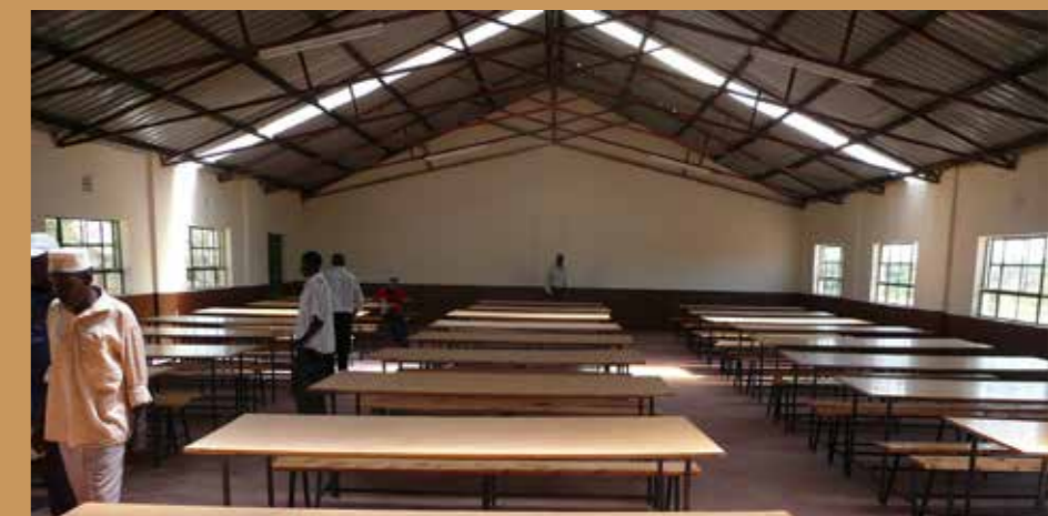
The new dining hall at Kilimani School, near Lewa's northern boundary.
